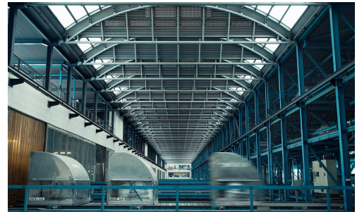
Inside Hactl’s massive automated Container Storage System.
