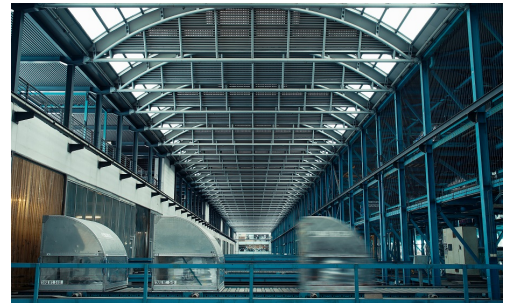
Inside Hactl’s massive automated Container Storage System.
